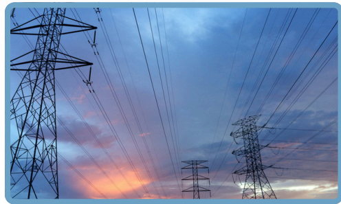
Power & Energy (Smart Meters)
